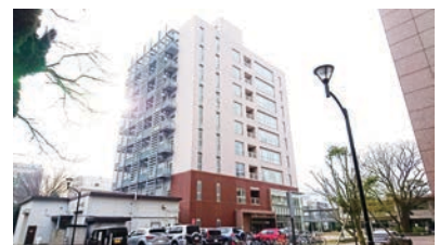
工学系総合研究棟2 Engineering Research Building II
